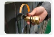
4. Connect the natural gas hose to the natural gas supply line.
