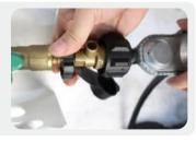
6. Turn the LPG tank valve to the fully open position.
